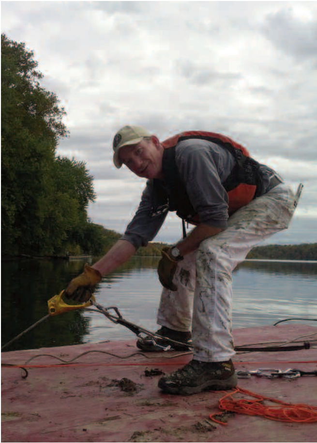
Joe Hage using a rock climbing ascender and carabiners to raise the anchors on the swim float
