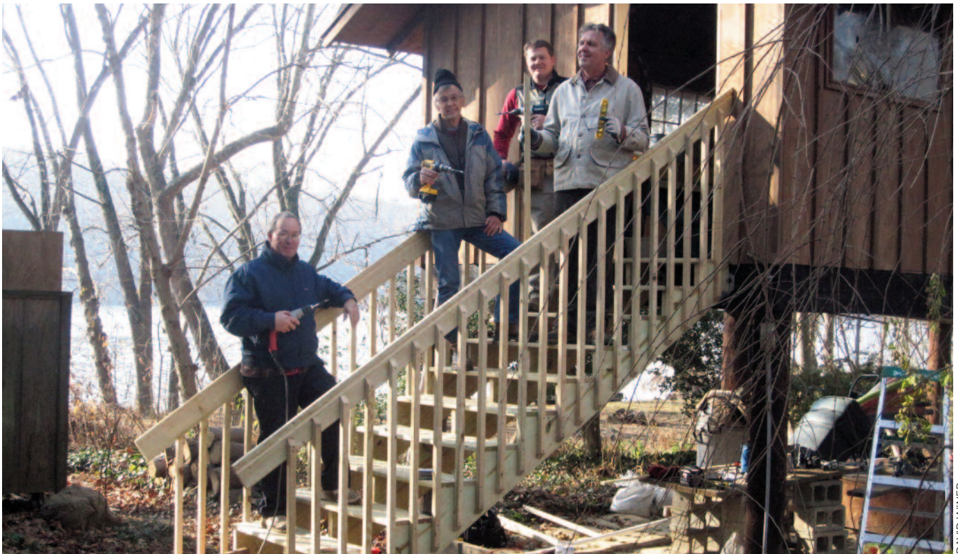
New stairs to the shed.
