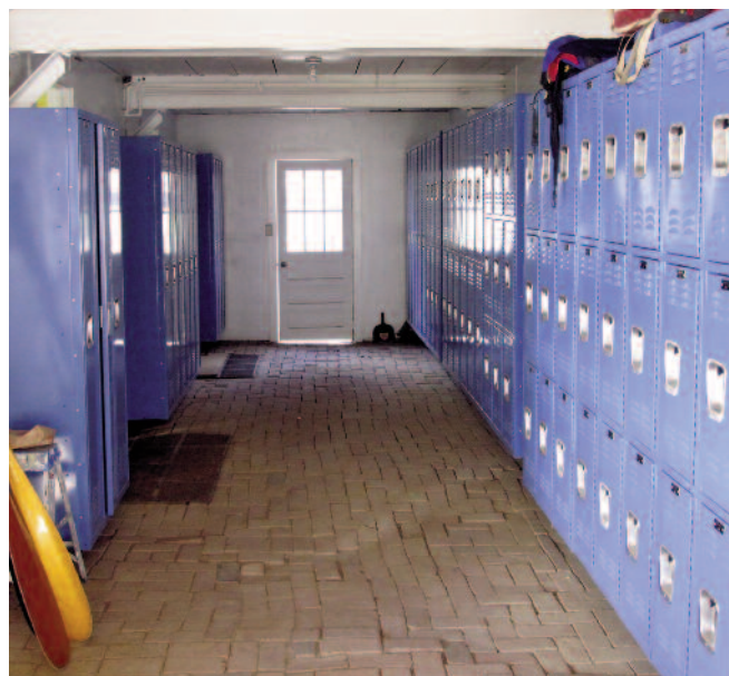
The installation of lockers is now complete.
