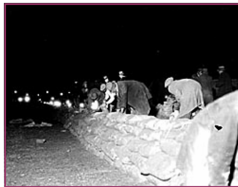
Washington, D.C., March 19, 1936; WPA workmen erecting emergency flood levee
