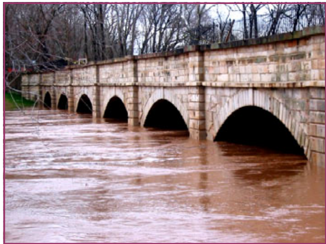
The Monocacy Aqueduct
