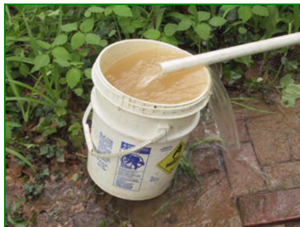
A day of pumping water out was needed to clear the clay from the loads of gravel placed in the well.
