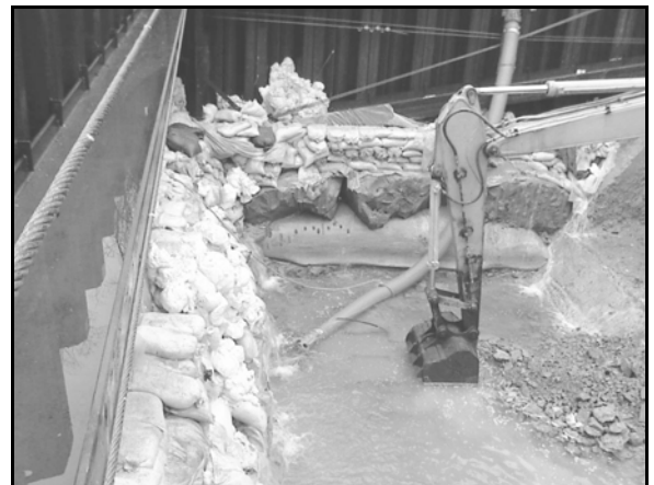
Digging from the river bottom in the fishway notch.
