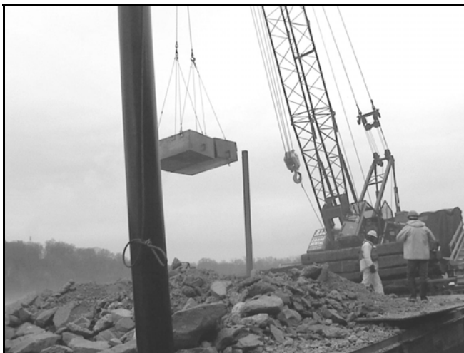
Buckets of old dam material are transferred to barges.
