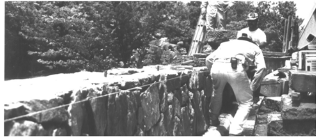
Placing cap-stones recycled from old wall.
