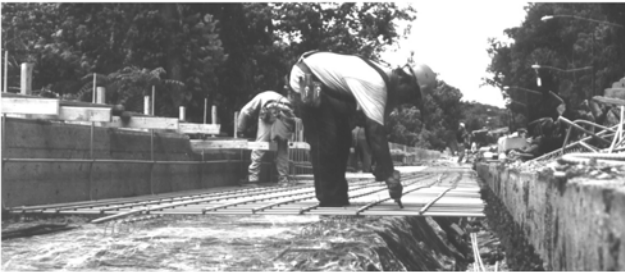
Laying reinforcing bars under new roadbed, next to wall.
