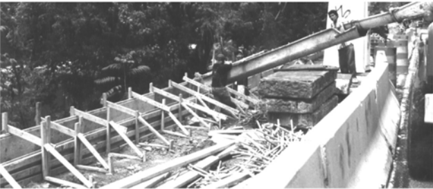
Pouring new foundation on old wall's sub-level.
