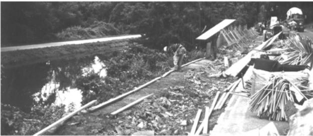
Upper layer of old wall removed.
