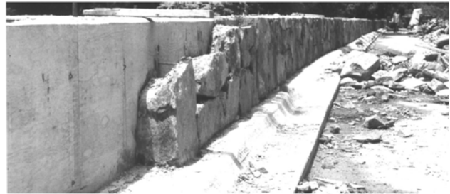
Inner wall finished, adding facing stones recycled from old wall.
