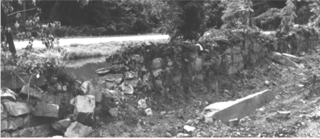
Digging the roadbed away.
